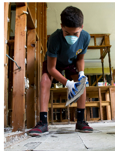
A 4-H'er wears a dust mask as he gathers damaged floor tiles on Aug. 27, 2016, at a home in Livingston Parish that was damaged when the area flooded earlier that month. Photo by Olivia McClure
