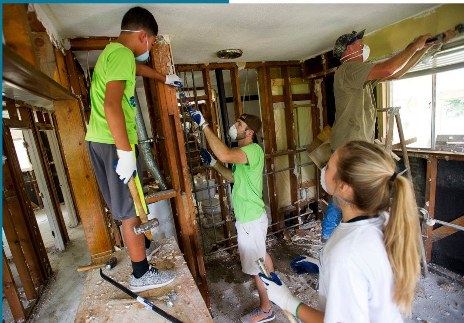
Cameron Parish 4-H'ers remove damaged materials from the kitchen of a Livingston Parish home that was damaged in historic flooding in August 2016. The 4-H'ers visited the parish on Aug. 27 to donate food they had collected and to help this homeowner begin the cleanup and recovery process. Photo by Olivia McClure
